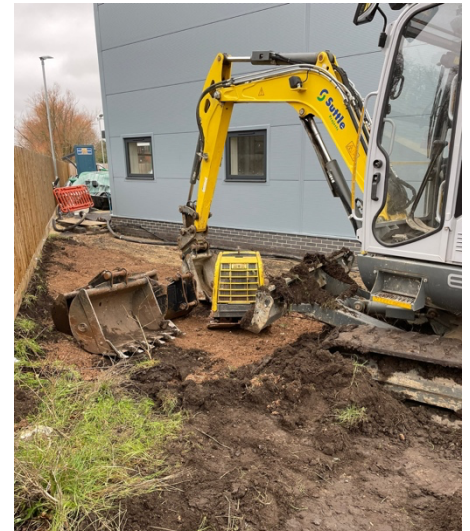
Figure 1: The small area in which the piling was to take place
